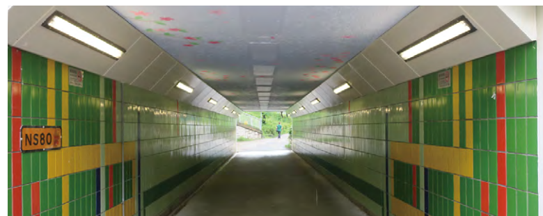
Subway at On Po Road near Tai Po Centre
