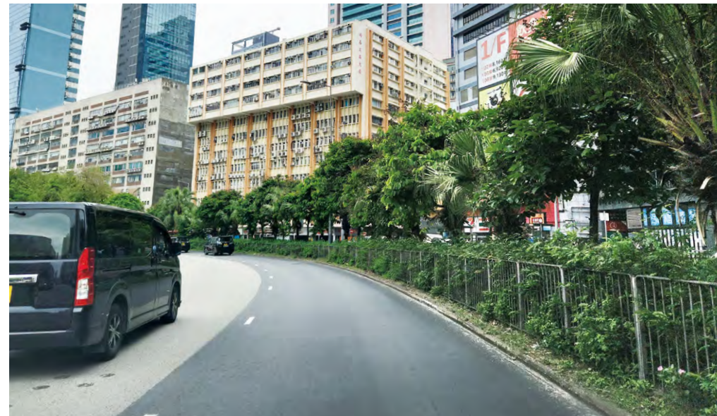
Rubberized bituminous pavement materials laid at Cheung Sha Wan Road
