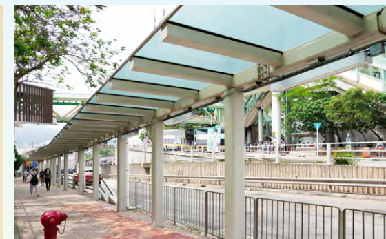
Walkway cover with laminated tempered glass panels
