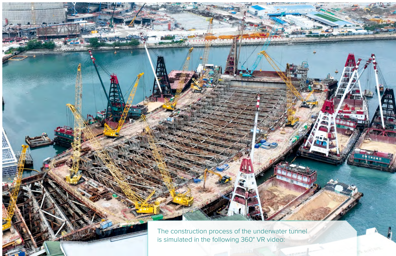
The underwater tunnel at Kowloon Bay under construction
