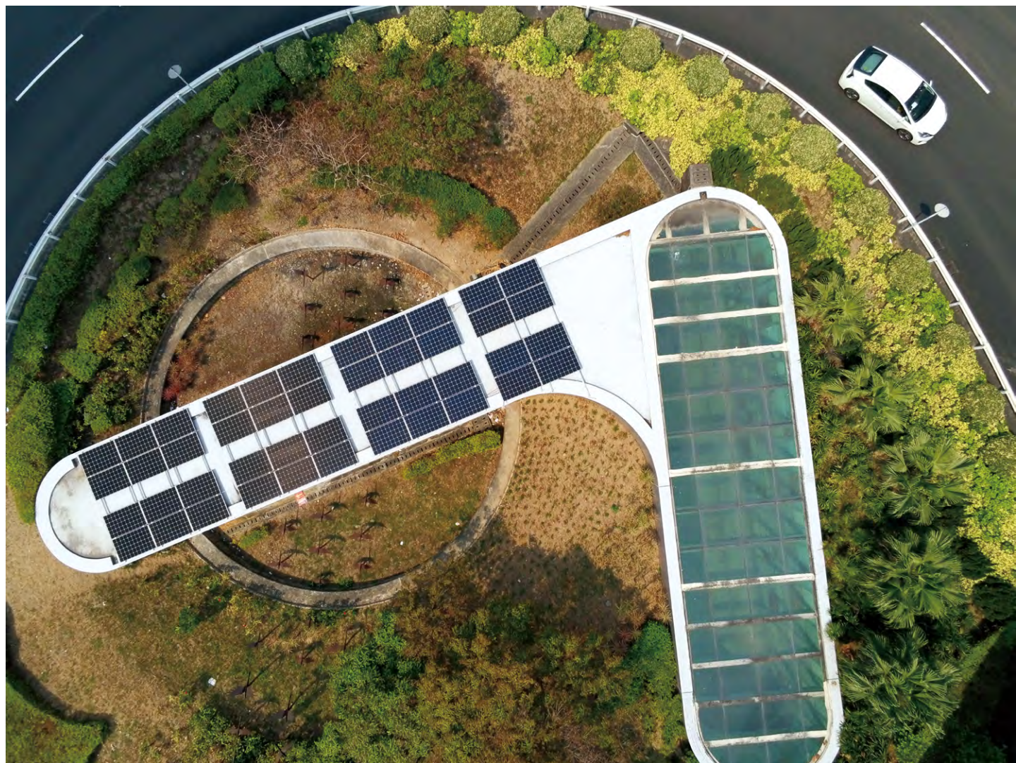
PV system on the roof of the existing subway at Kwai Fuk Road
