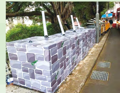
Tree support system with tree ties connecting to concrete blocks
