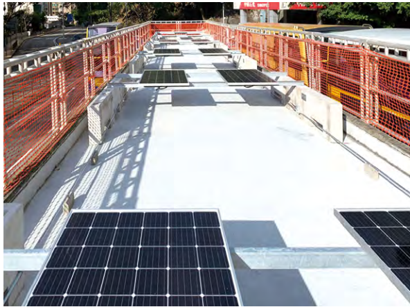
Subway at Pok Fu Lam Road near Pokfield Road (completed in 2020)
