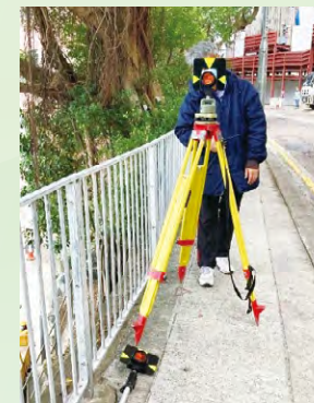
Monitoring survey to track tree displacement
