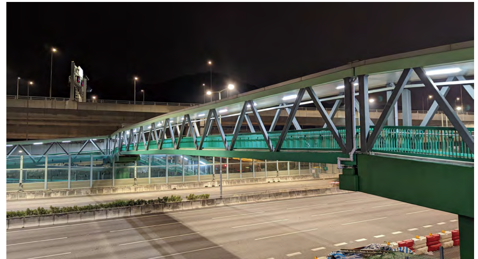
A footbridge with LED lights
