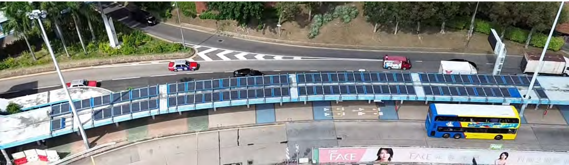
PV System at the covered walkway at Hong Chong Road near Hong Kong Polytechnic University
