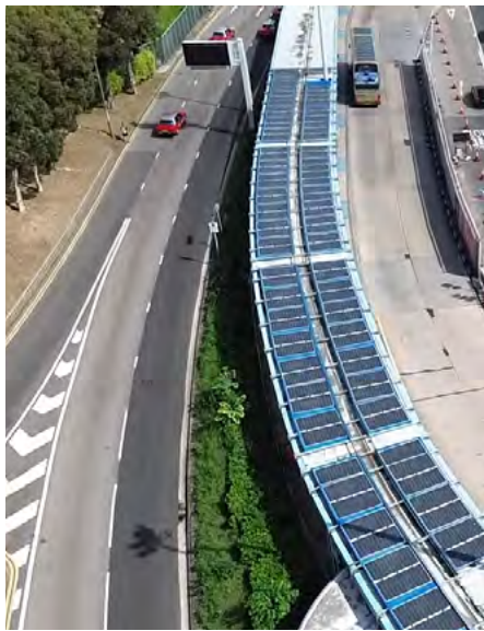
PV system at the covered walkway at Hong Chong Road near Hong Kong Polytechnic University
