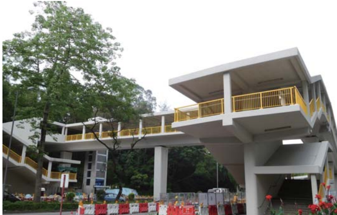
Provision of BFA facilities at footbridge across Ting Kok Road
