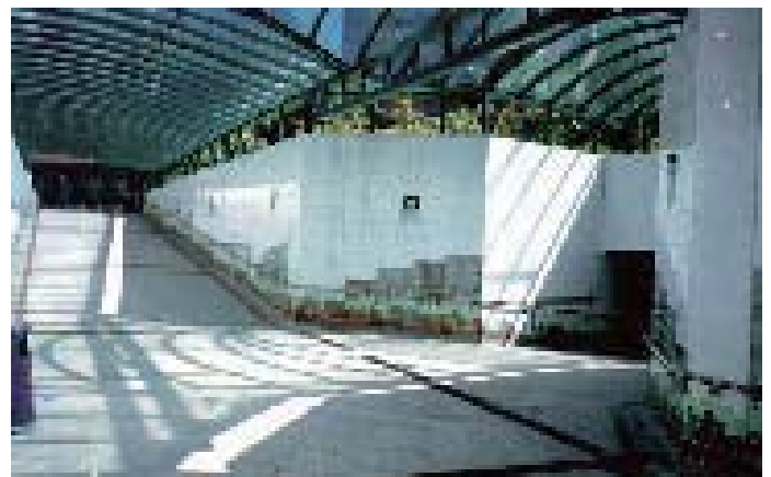
Forecourt Subway across Sports Road at Happy Valley
