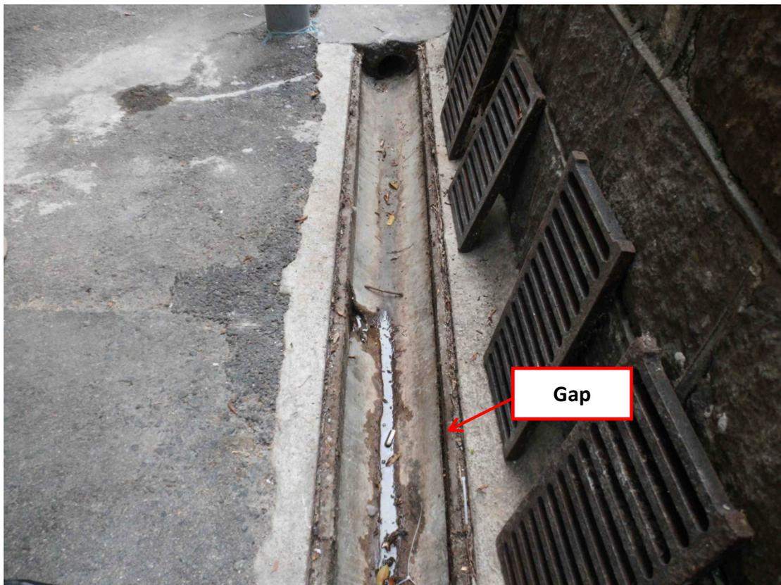
**Record of longitudinal gap found along the back of coping of stonewall near tree T1 and transverse crack through the same coping**
