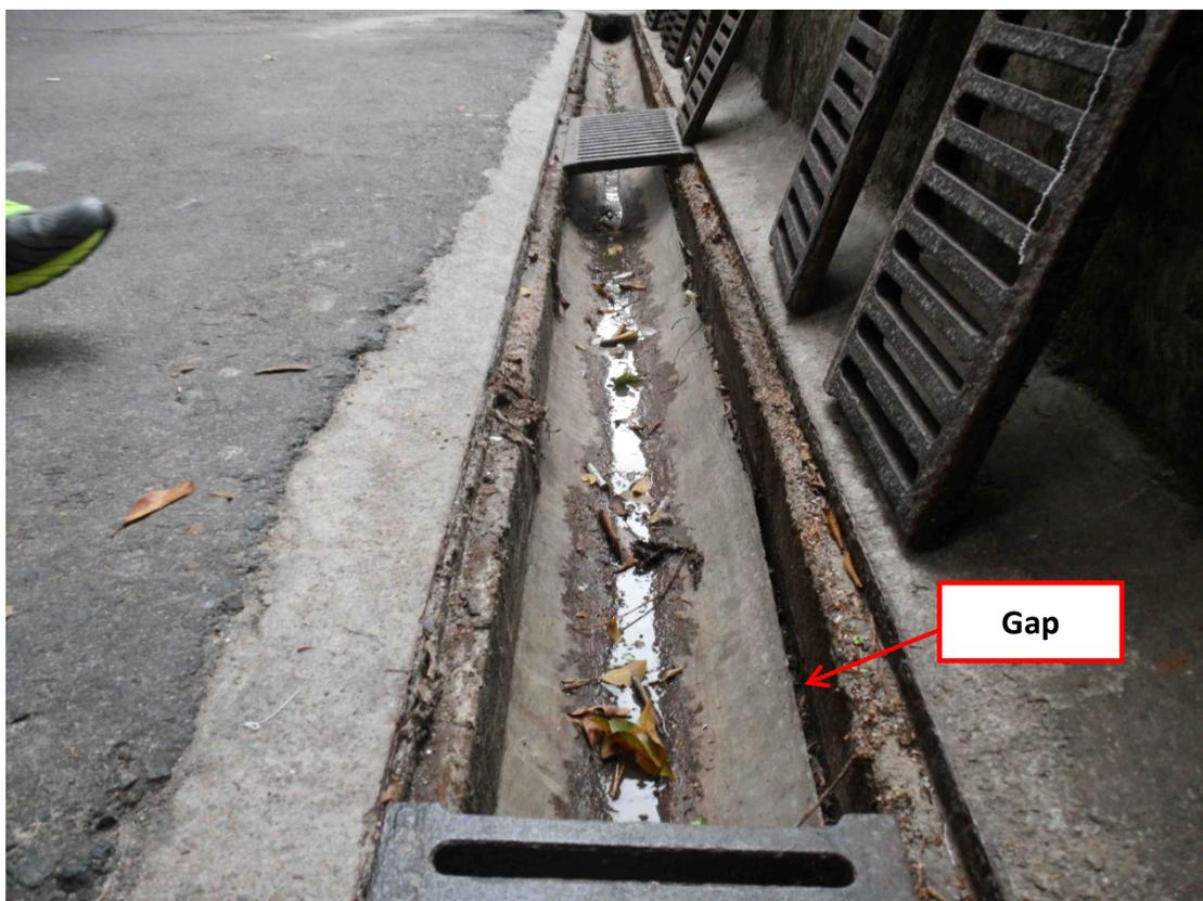
**Record of 15mm wide longitudinal gap found along the side of a U-channel at the coping of stonewall**
