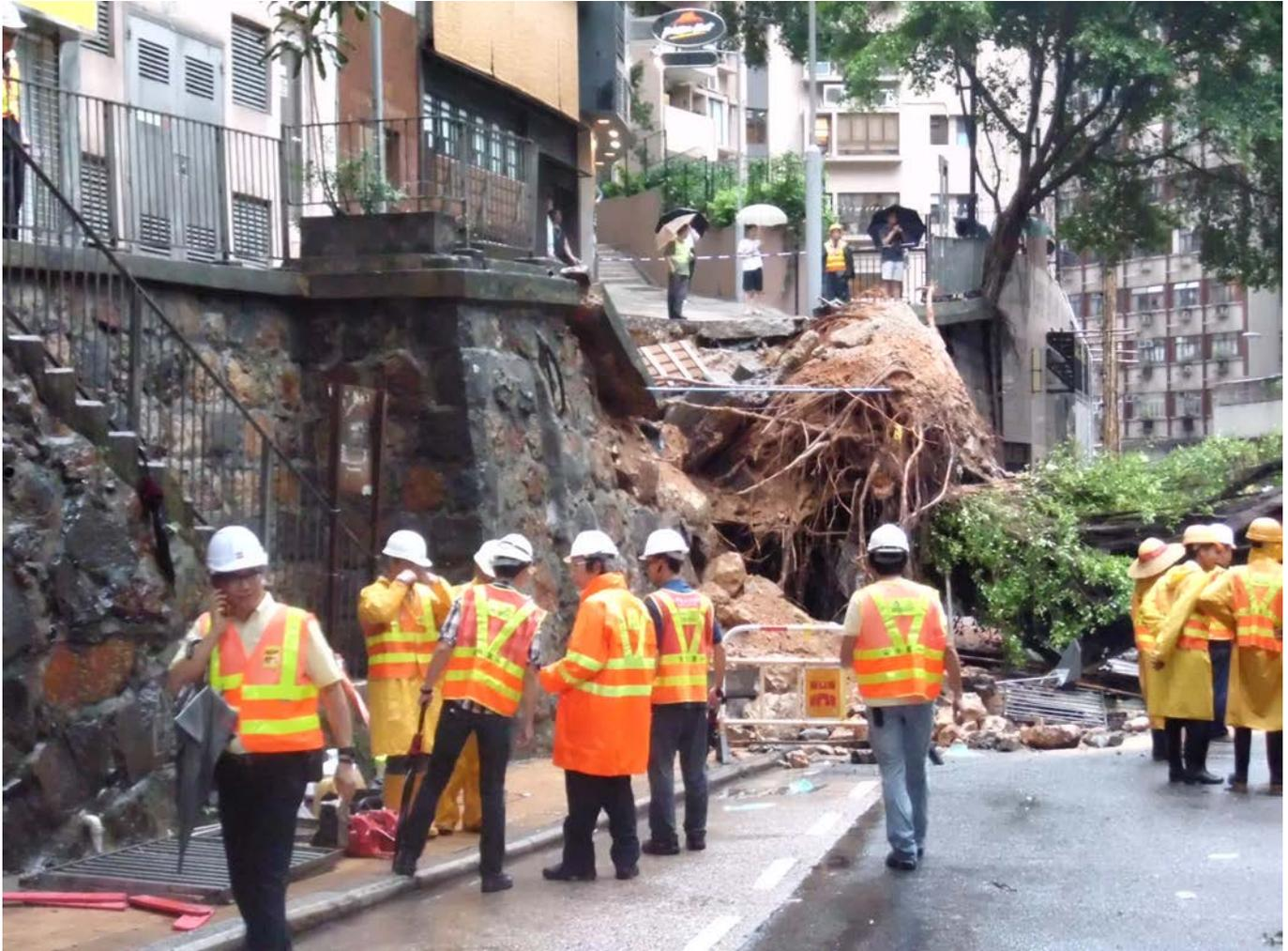
Photo 2.2 – Stonewall Damaged together with Tree T2
