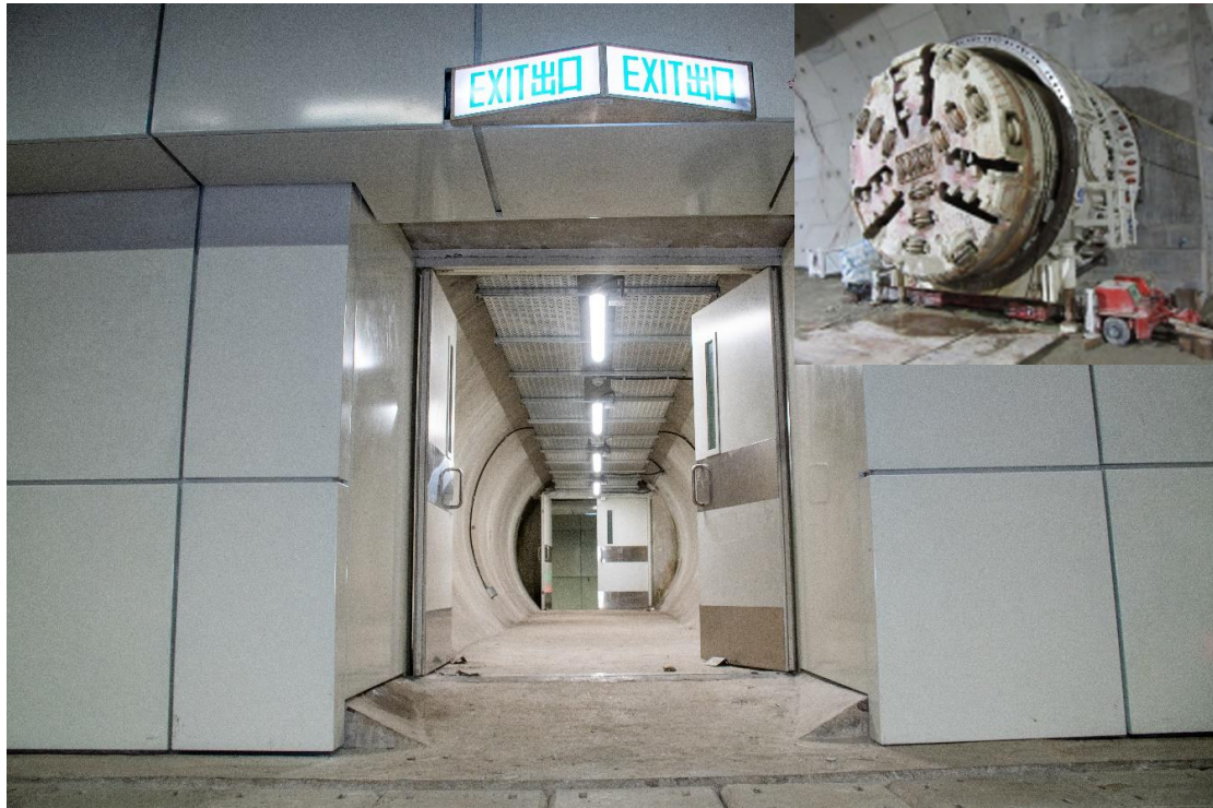
Breakthrough of Mini-Tunnel Boring Machine at Cross Passage
