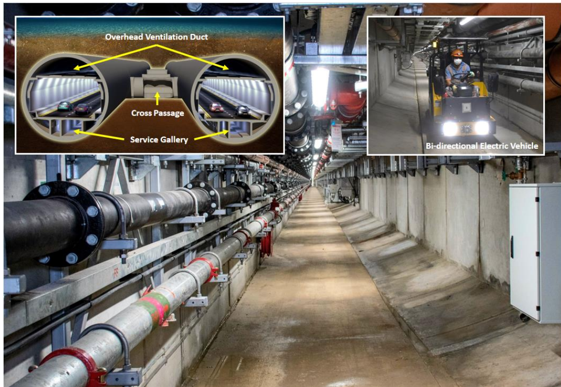
First Sub-sea Tunnel with Service Gallery for Electrical and Mechanical Installations in HK
