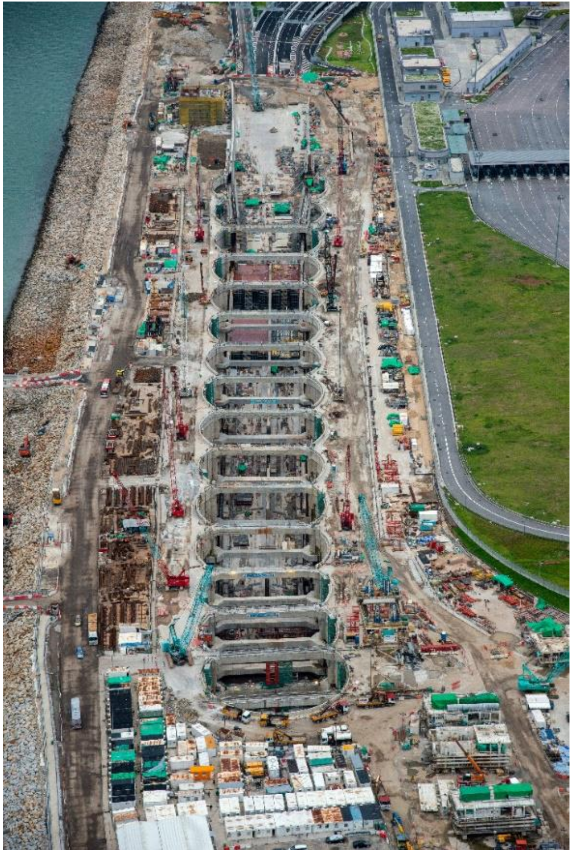
Largest Caterpillar Cofferdam Structure in Hong Kong – Cut and Cover Tunnel at Southern Landfall
