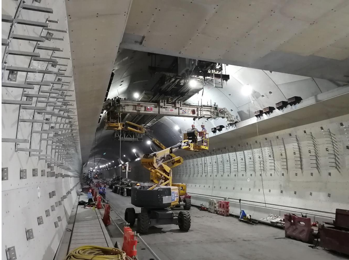
Assembling of Precast Slabs for Overhead Ventilation Ducts inside Tunnel
