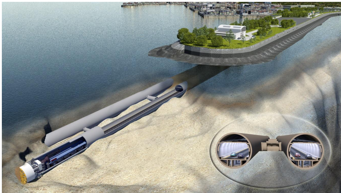
First Sub-sea Road Tunnel in Hong Kong Constructed by TBM
