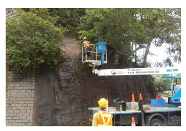
Cleaning blocked weepholes and repairing cracked surfacing on a roadside slope
