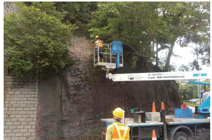
Cleaning blocked weepholes and repairing cracked surfacing on a roadside slope
