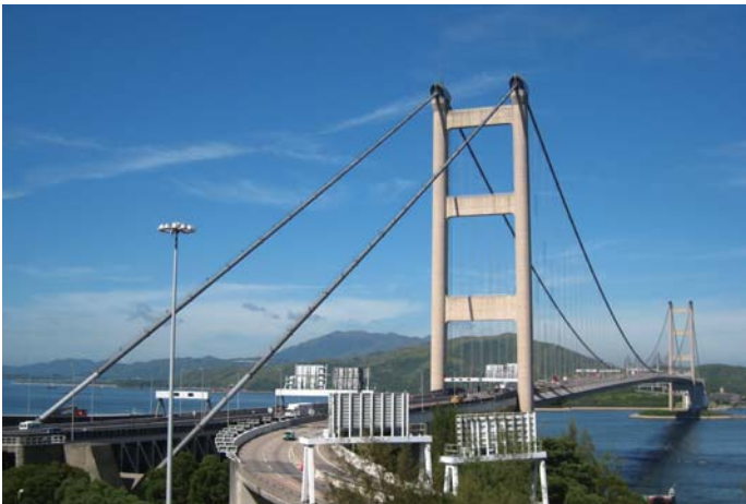
Tsing Ma Bridge
