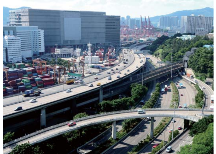
Kwai Chung Viaduct
