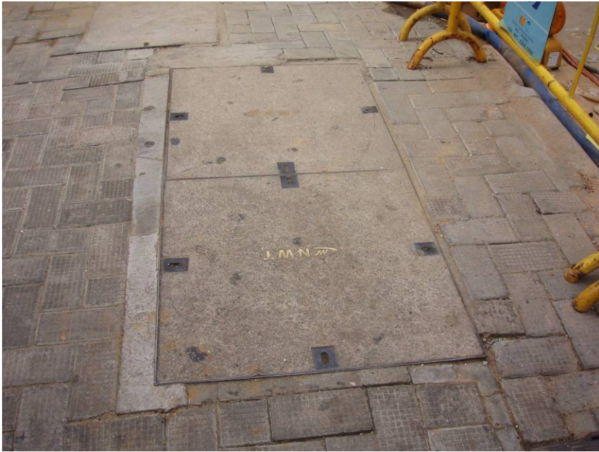
Photo 3 -- Joint Chamber (Concrete Cover Type—NWT)
