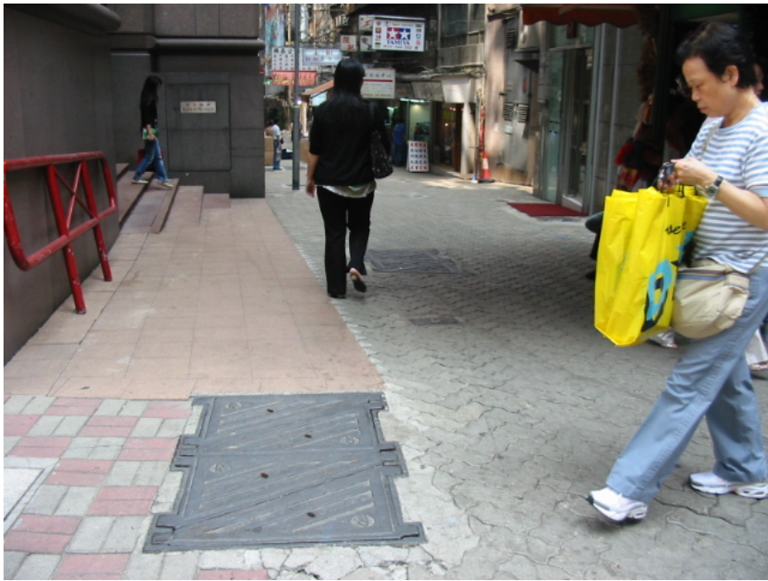
Photo 4 -- Joint Chamber Heavy Duty Cover Type—NWT)
