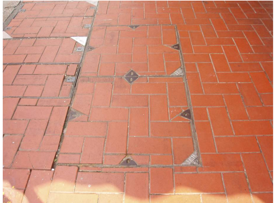
Photo 4 -- Joint Chamber (Recess Cover Type—NWT)
