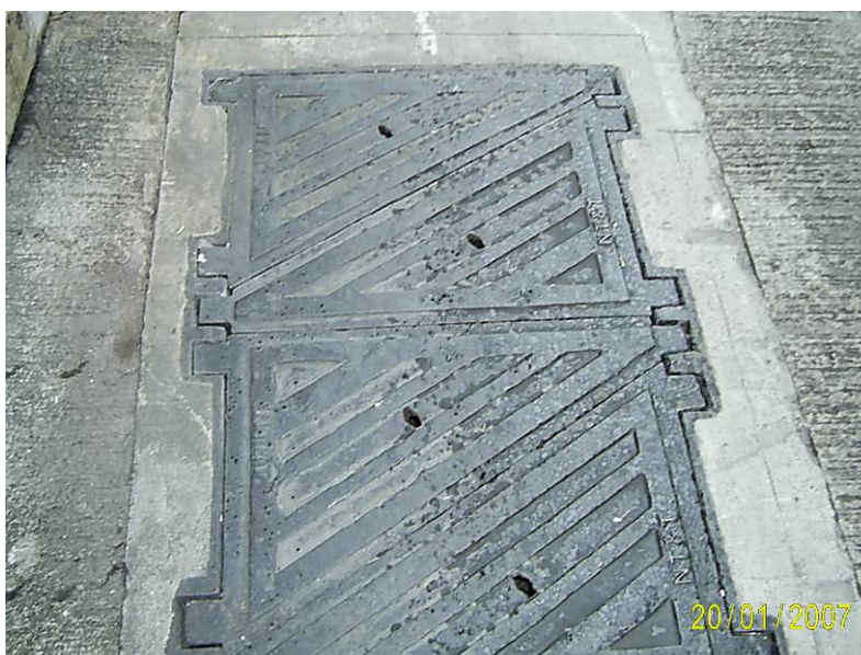
Photo No.2 (Manhole/Joint Box- Carriageway Type) Covers Number: From 1-6
