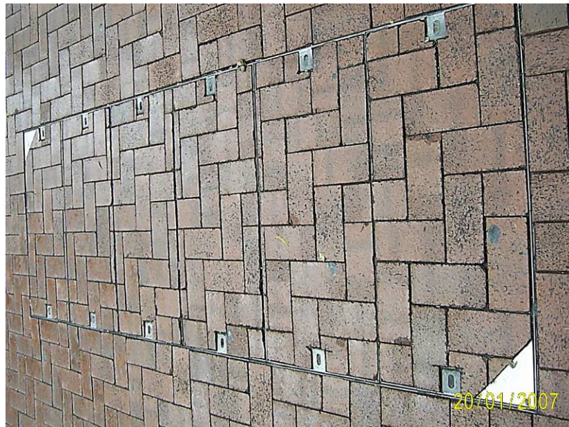
Photo No.4 (Manhole/Joint Box- Recessed Type) Covers Number: From 1-6
