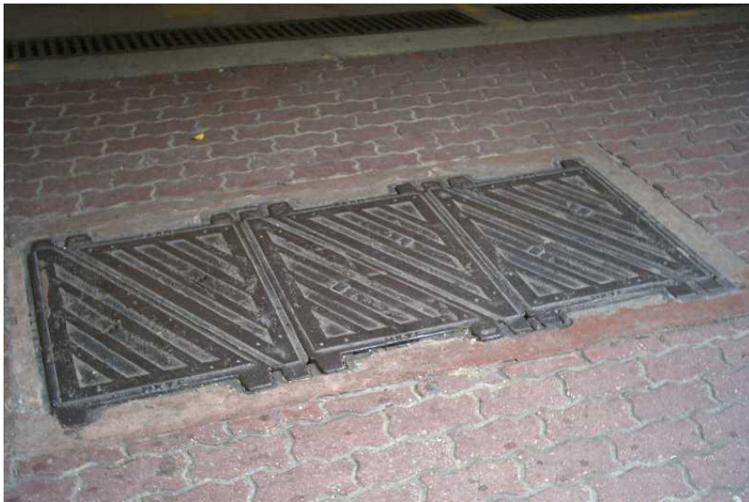
Photo No. 9 (Manhole/Joint Box – Carriageway Type) Covers Number : from 2-6
