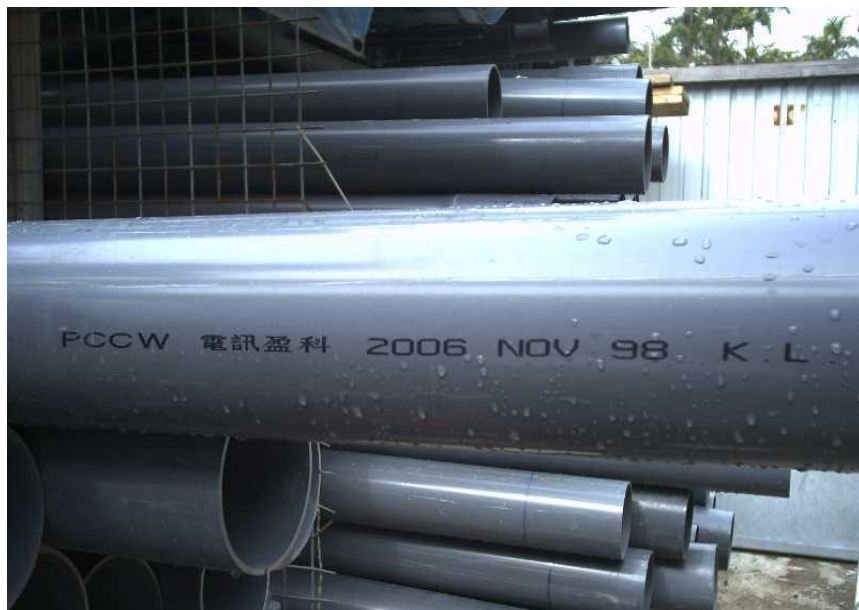
Photo No. 1 (PVC Duct : Diameter 30-107mm) Buried at Depth : 450mm
