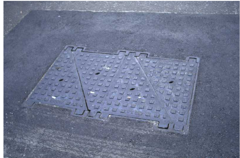
Photo No. 10 (Manhole/Joint Box – Carriageway Type) Covers Number : from 2-6
