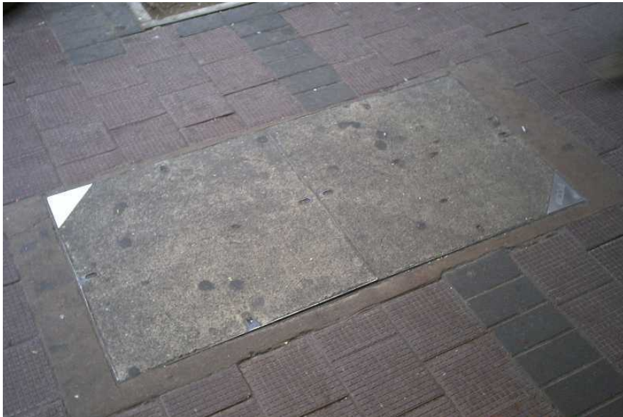
Photo No. 7 (Manhole/Joint Box – Concrete Type) Covers Number : from 1-3
