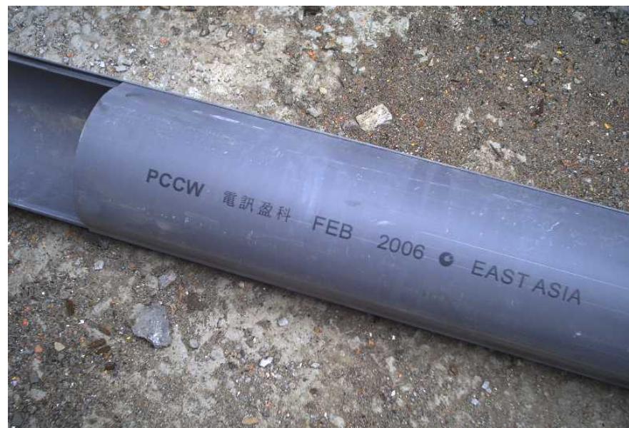
Photo No. 2 (PVC Split Duct : Diameter - 107mm) Buried at Depth : 450mm
