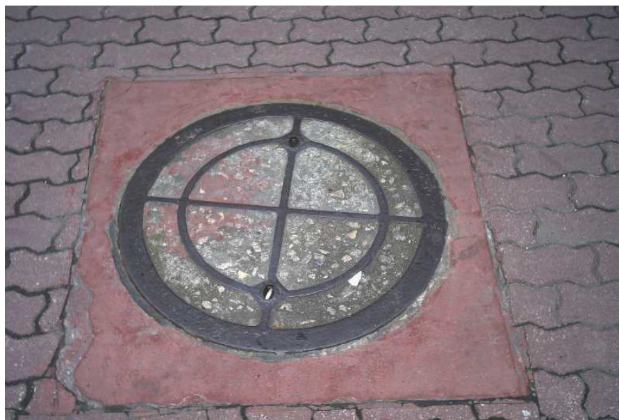
Photo No. 11 (Manhole – Carriageway Type) Circular Cover
