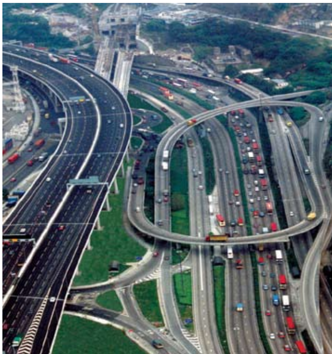
Kwai Chung Viaduct
