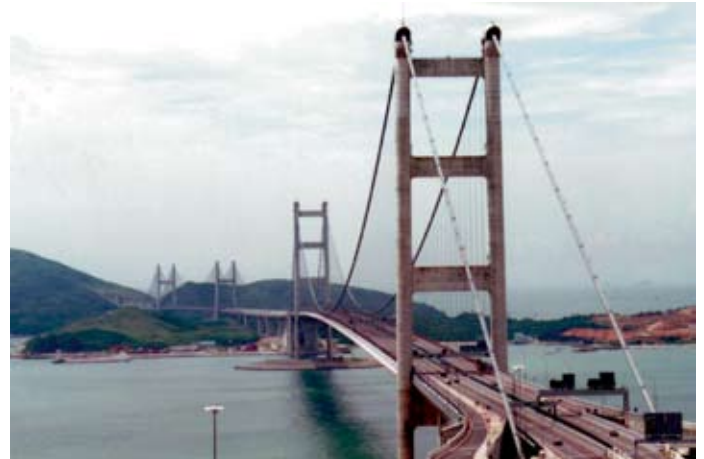
Tsing Ma Bridge
