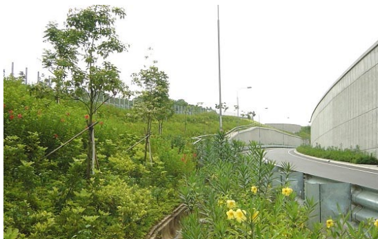
Planting for slope greening
