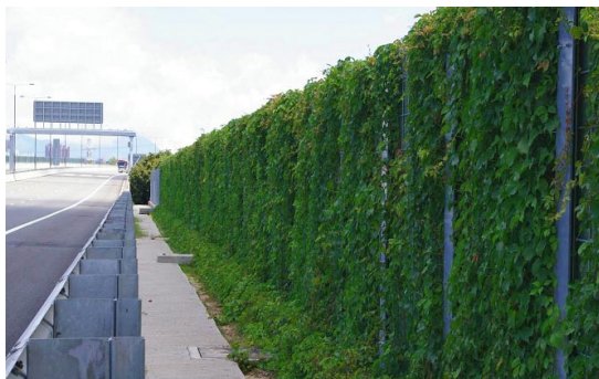
Planting adjacent to noise barrier
