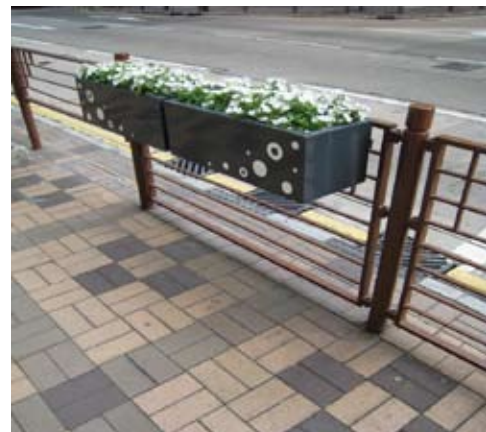
Upgraded paving and road side hanging planter along Canton Road
