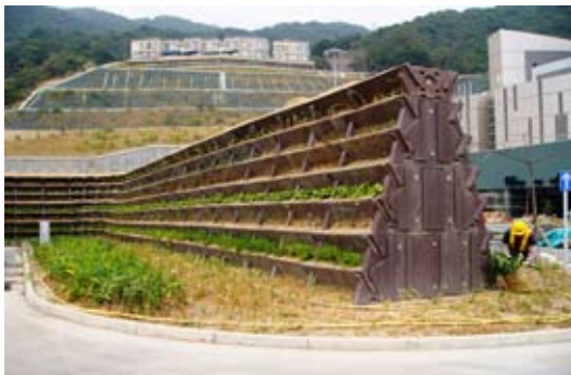
Route 8 engineered earth mound
