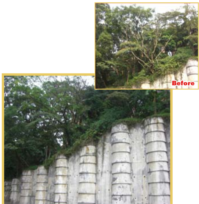
Horticultural maintenance – removal of dead tree
