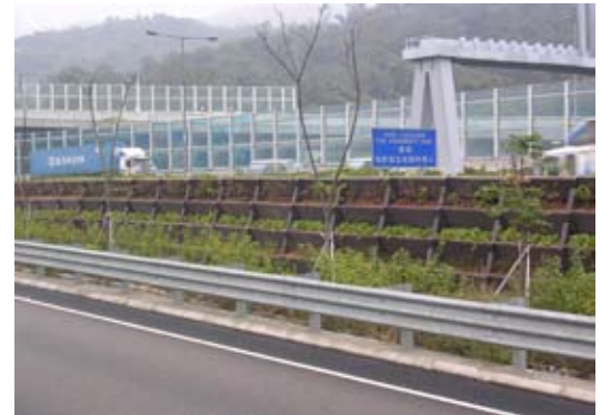
Earth mound along Yuen Long Highway north bound to Kong Sham Western Highway north bound
