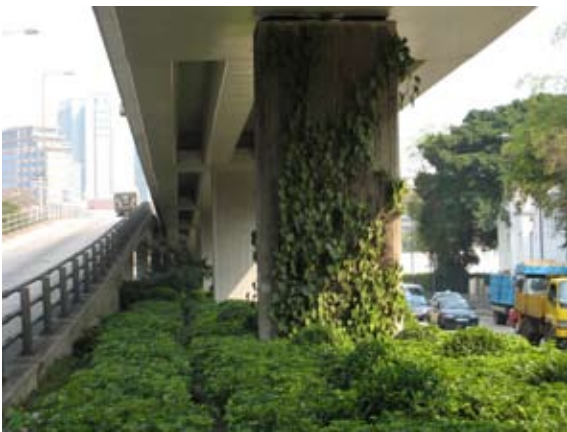
Greening along Gascoigne Road Flyover
