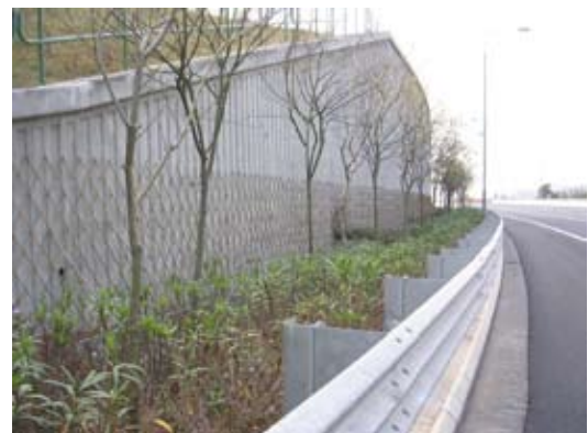
The climbing system along Kong Sham Western Highway north bound near Ngau Hom Shek
