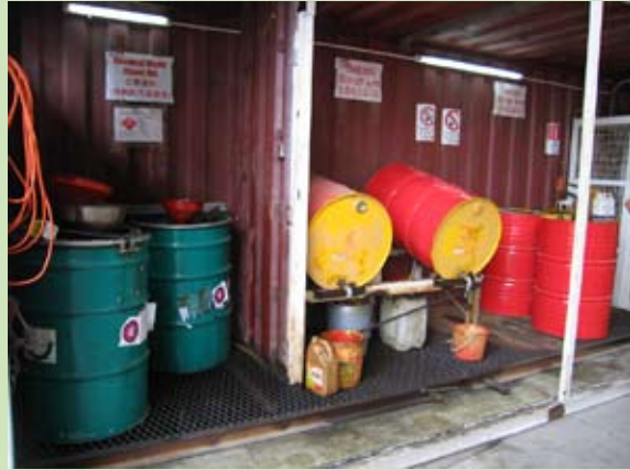
Storage of chemical waste to avoid work site contamination
