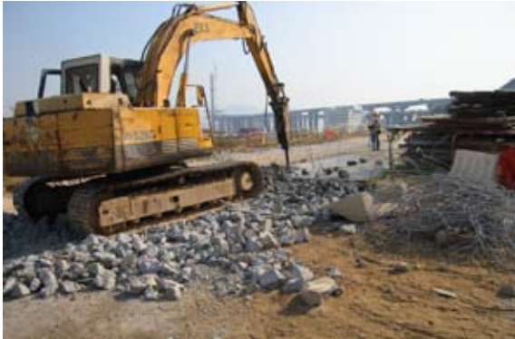
Recovery of steel reinforcement bars from broken concrete
