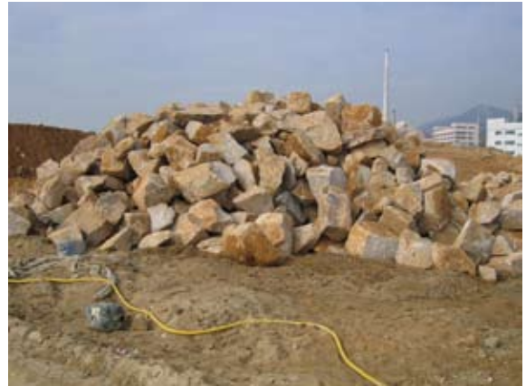
Sorting out of good quality granite from cut-slope work for reuse
