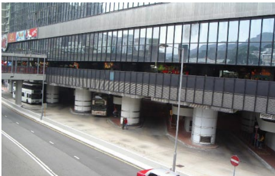
Fan schedule of the PTI at Nan Fung Centre has already been adjusted to achieve energy saving
