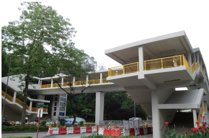
Provision of BFA facilities at footbridge across Ting Kok Road
