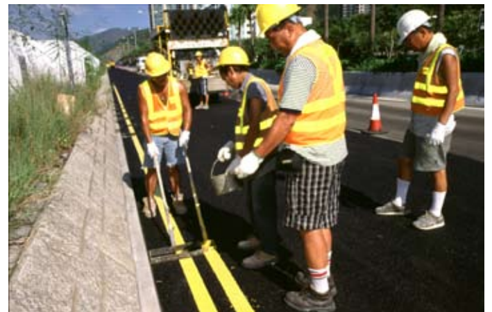
重髹道路標記 Road marking repaint
