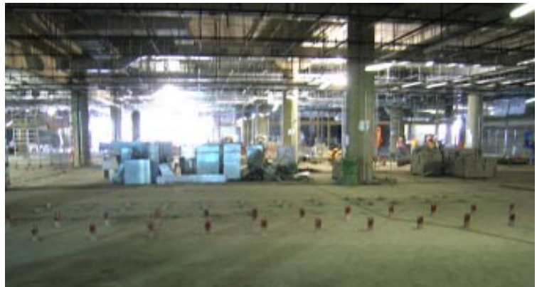
Internal building works at the future departure hall
