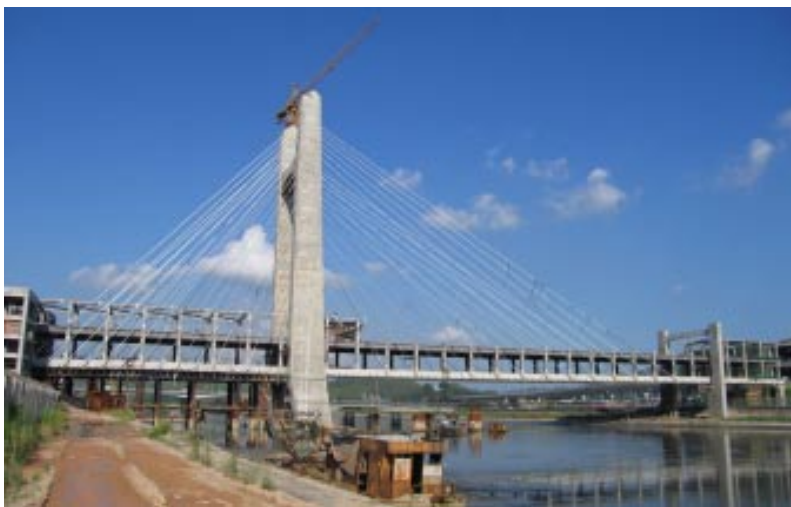
Passenger Bridge deck structure construction
