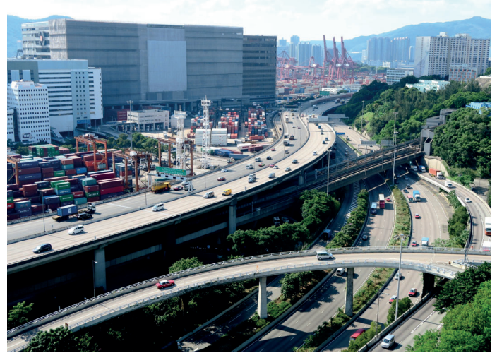
Kwai Chung Viaduct
