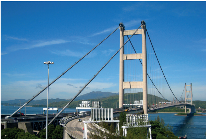
Tsing Ma Bridge
